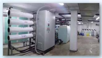
Desalination plant, daily capacity 80m³ of drinking water, installed in hotel Nikki Beach 5\*, in Porto Heli.
