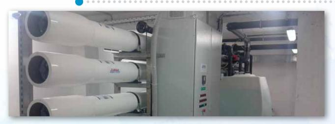
**TEMAK** designed and manufactured the new control panel **RO-T4** for desalination plants with reverse osmosis, to replace the previous model RO-T3.
